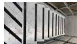
383 La Trobe St, Melbourne - Emergency Stair
