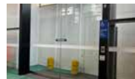
664 Collins St, Melbourne - DDA Door to Lobby
