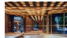
124 Exhibition St, Melbourne - Services Replacement & Lobby
