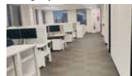
90 Collins St, Melbourne - Investigative Structural Works & Reinstatement
