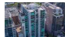
Aurora Apartments, Melbourne - Recladding Works
